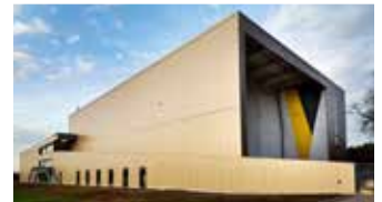
MONTANATHERM® Kletterhalle, Uster (CH)
