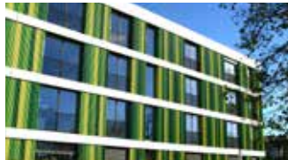
MONTAFORM DESIGN® Widmi, Lenzburg (CH)
