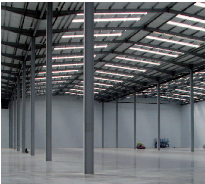
Test building with Colorcoat® PE 15 internal liner and Colorcoat® High Reflect.
