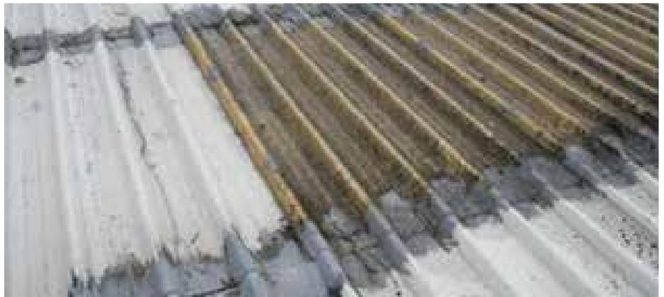
Figure 16. Before refurbishment showing failed roof cladding
