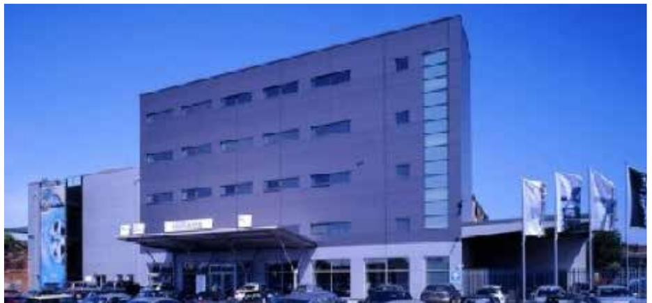
Figure 22. Building after pre-finished steel rainscreen over cladding system
