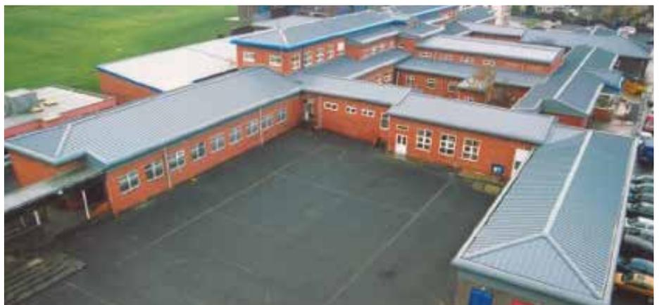
Figure 19. School after pre-finished steel flat to pitch roof system refurbishment
