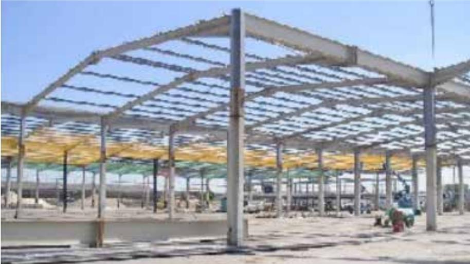
Figure 6. Refurbished portal frame ready for re-sheeting
