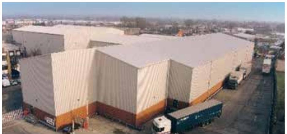
Figure 15. Refurbished building after pre-finished steel roof over cladding and the inclusion of improved insulation
