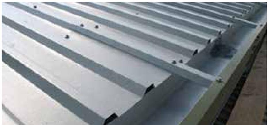
Figure 17. Roof after refurbishment showing pre-finished steel composite panel roof cladding
