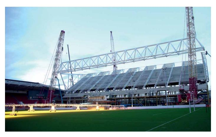
arrangement of chords and braces – overlaid with aesthetic considerations – which posed a complex challenge for the most complicated joints and loading calculations. It was very satisfying to be able to assist J&D Pierce in reaching a satisfactory solution."
