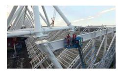
most arduous conditions. The consistent strength and tolerance delivered by Celsius 355 were important factors in the successful design and fabrication of the bespoke truss arrangement. Throughout the detail design phase, Tata Steel's Customer Technical Services team was on hand to assist with the design of complex welded joints.
