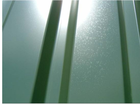
Visible effect: thin, white deposit (fig. D1 and D2)
