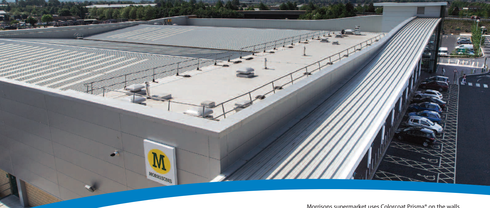
Morrisons supermarket uses Colorcoat Prisma® on the walls and Colorcoat HPS200 Ultra® on the roof.
