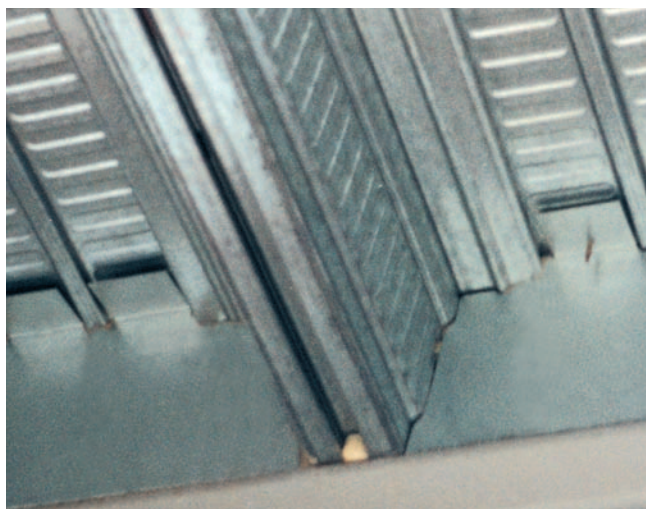
Figure 1.3 Diaphragm fixing
