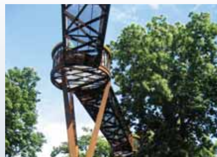
Xstrata Aerial Walkway, Kew Gardens (photograph: Jane Wernick, Jane Wernick Associates)
