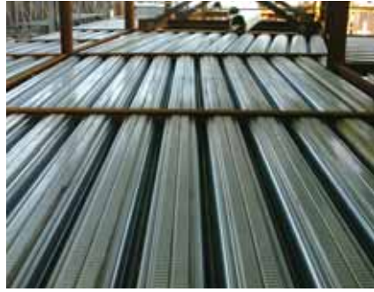
The Slimdek flooring system is a result of extensive research and development work
