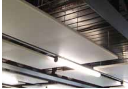
Interior of Bridge Academy, Hackney, showing exposed composite flooring
