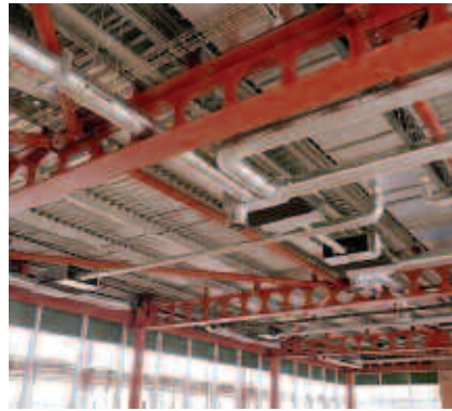
Service integration within cellular beams.
