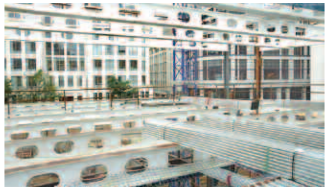
Long-span cellular beams.
