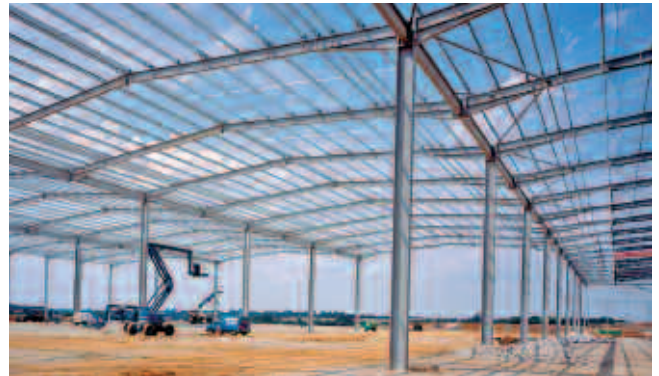
Long-span structural frames.
