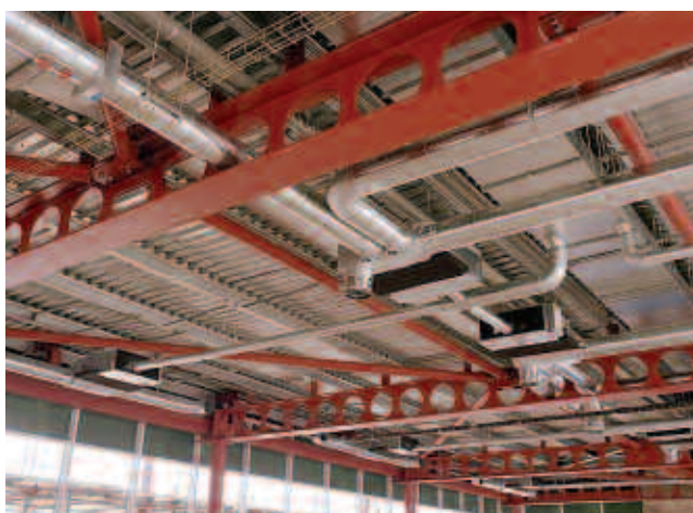
Service integration within cellular beams.
