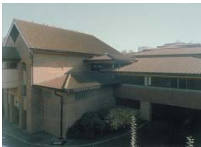
Figure 18. Guildford 946 space Car Park adjacent to railway and local housing
