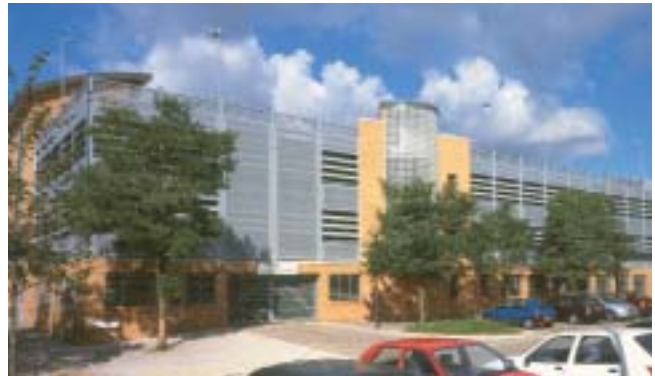
Figure 23. Avebury Boulevard multi-storey car park, Milton Keynes.
