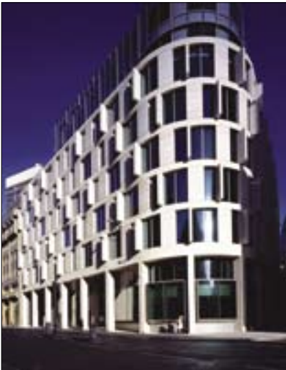
Figure 62 Plantation Place South: an office building in the centre of the City. An advanced fire analysis demonstrated that much of the steelwork could be left unprotected.
