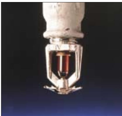
Figure 10 Typical sprinkler head configuration. The red colour of the volatile liquid indicates that the glass will break at 68°C. This is the most common activation temperature.
