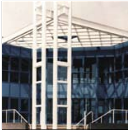
Figure 20 Intumescent coated hollow sections. Courtesy of Carboline Ltd.
