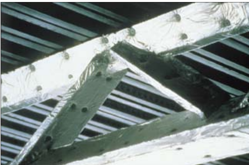
Figure 26 Flexible blanket protection system.
