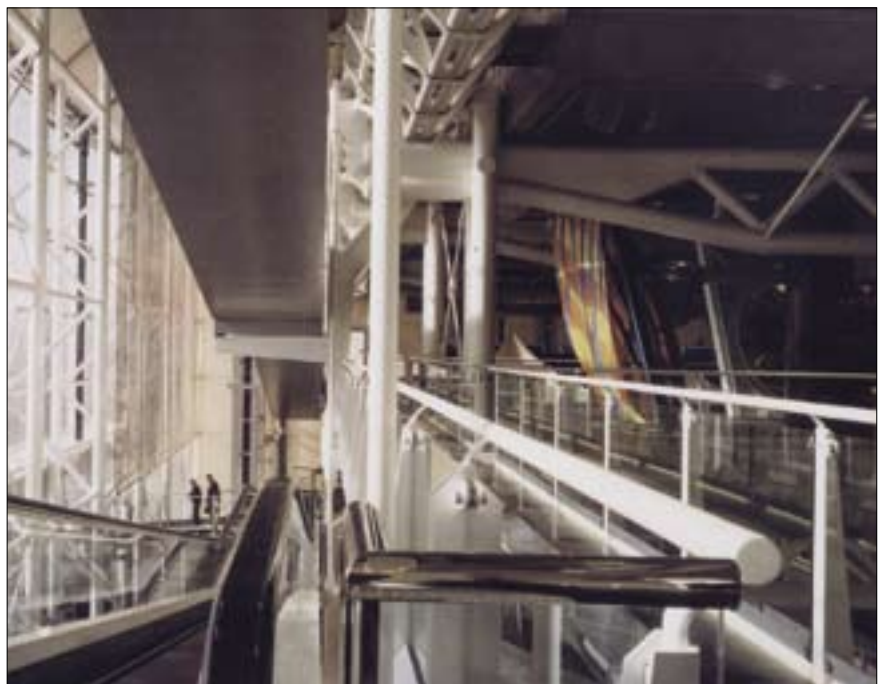
Figure 25 The British Pavilion at the Seville Expo. Structural fire protection with thin film intumescent coating. Courtesy of Leigh's Paints.
