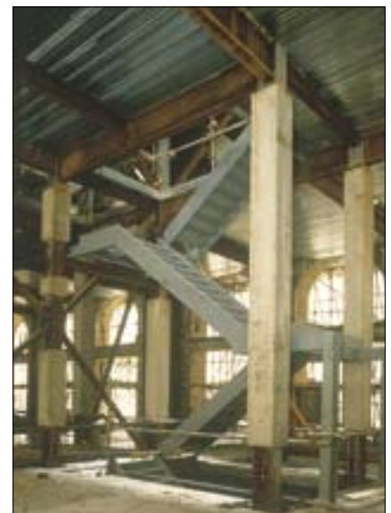
Figure 27 Concrete encasement.
