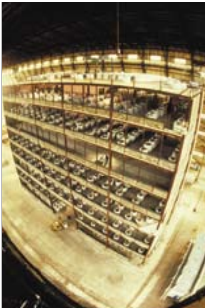
Figure 56 The Cardington frame is a multi-storey composite structure, i.e. the floors are constructed using shallow composite slabs with profiled steel decking attached by shear connectors to downstand beams. The design guidance developed from the fire tests applies only to frames of this type.
