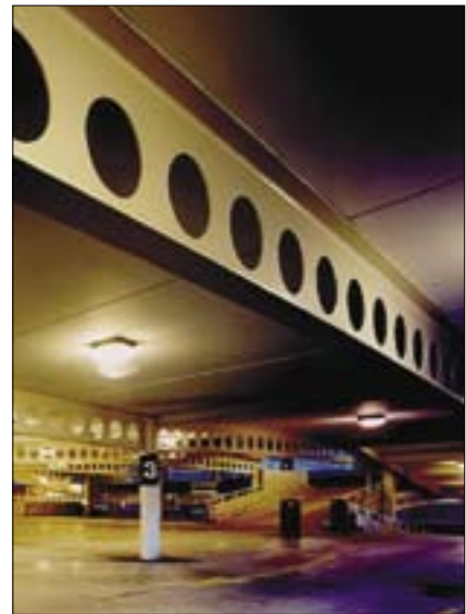
Figure 4 Steel in open deck car parks is usually unprotected.
