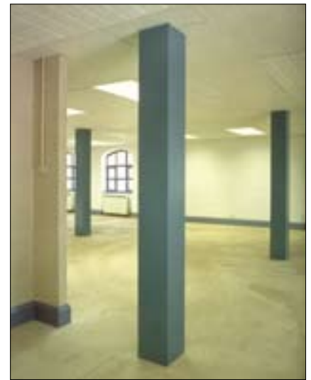
Figure 22 Board protection systems. Courtesy of Promat Ltd.
