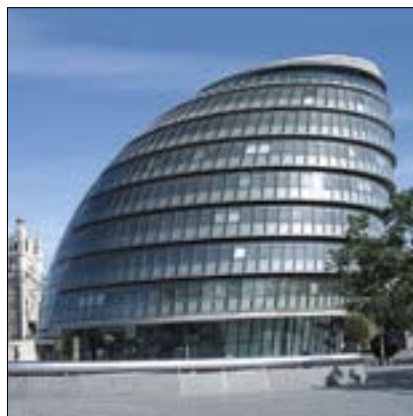
Figure 54 GLC building in London.
