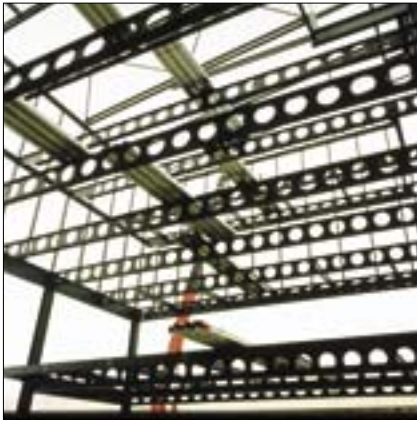
Figure 19 Cellular beams used at Lincoln University.
