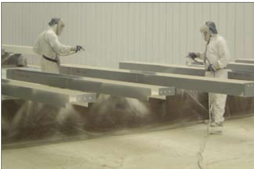
Figure 28 Manual application of off-site intumescent coatings.
