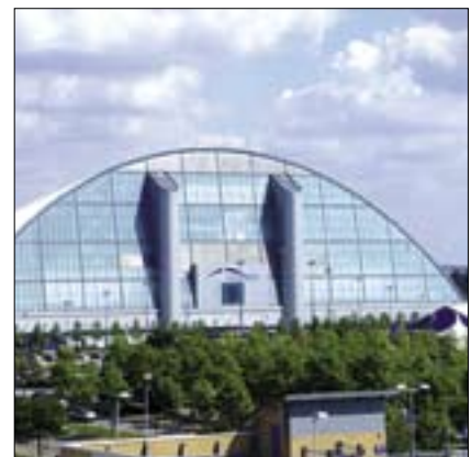
Figure 55 XSCAPE building in Milton Keynes.
