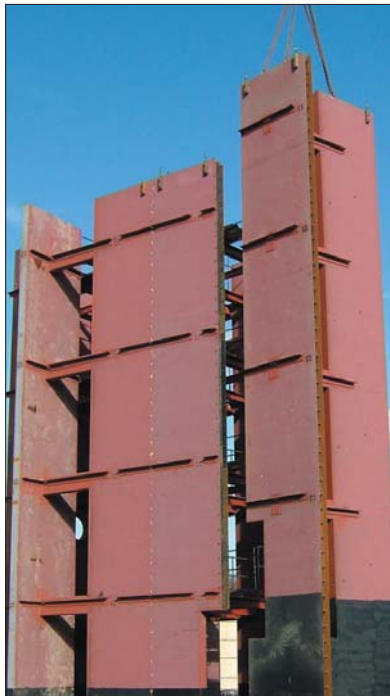
Right: Corefast is an innovative, off-site construction product for the rapid creation of structural cores in multi-storey buildings
