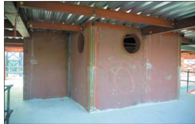
Right: Central Corefast core showing steelwork, floor decking and preform openings
