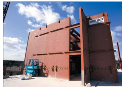
Left: Corefast central core showing pre-formed doorways and adjustable screw levelling
