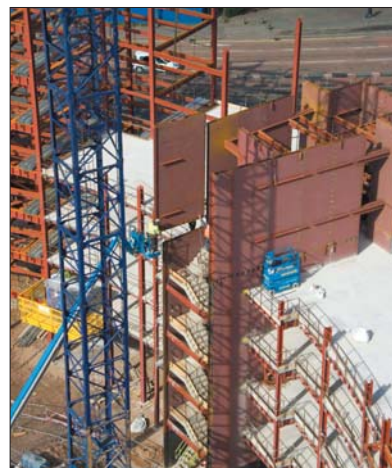
High level view of the site illustrating the central core with the prefabricated stairways installed up to the fourth level
