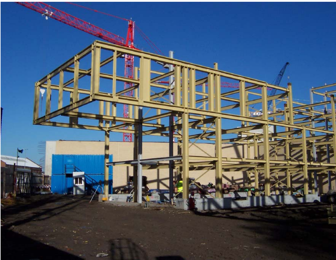
Photo: Courtesy of Billington Structures Ltd.
