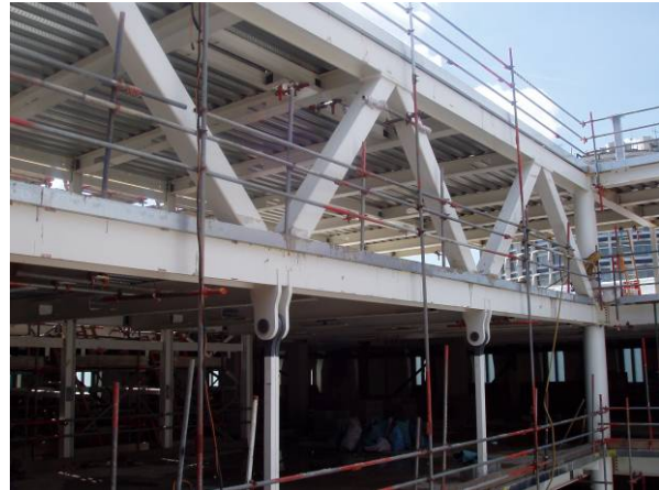
Floors hung from long-span steel truss
