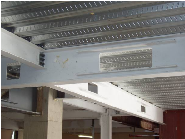
New steel structure with service routing
