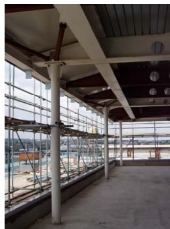
Columns at top floor
