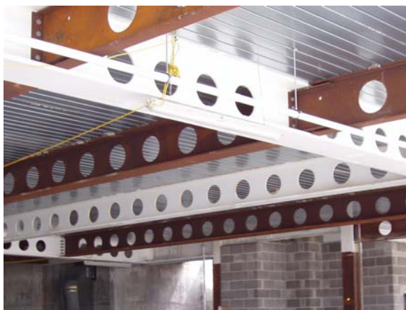
Intumescent coating applied to beams
