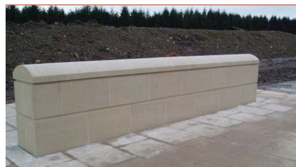
Above and right: Bi-Steel walls clad to provide discreet protection
